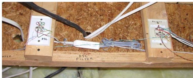
Here, the telephone service comes in on the left plate, office phone lines are on the right plate, and the DSL filter is connected between the two. The DSL modem line is wired to the left plate.
